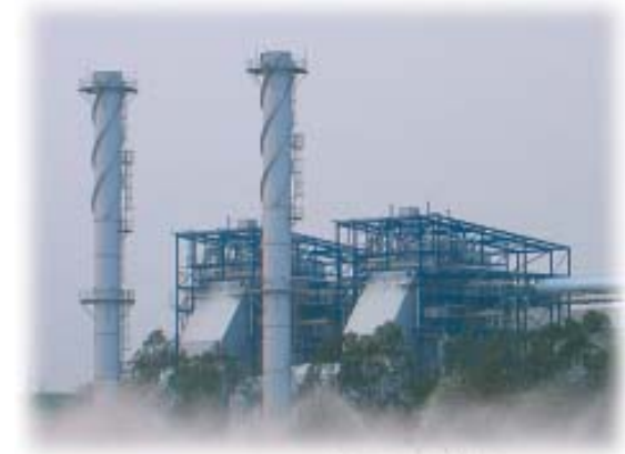
The 41 MWe bagasse-fired cogeneration plant
