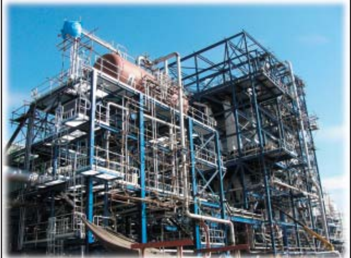
During erection of the cogeneration plant
