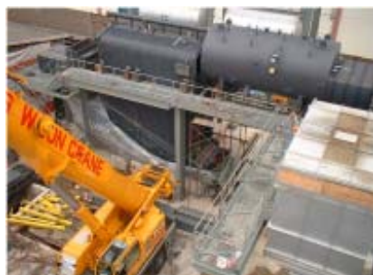
Cogeneration plant construction site
