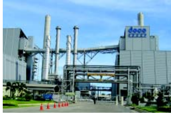
470 MW hybrid coal & gas-fired cogeneration plant, Thailand
